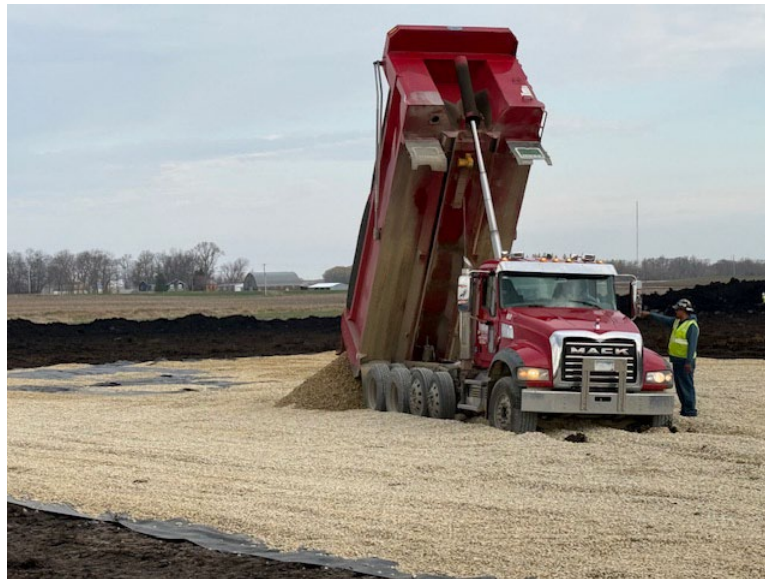
Facing northeast at MP 34.2, K&K dumping rock on geotextile for staging area north of 165th Street
