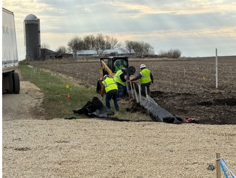
Facing east at MP 34.1, K&K installing ECDs
