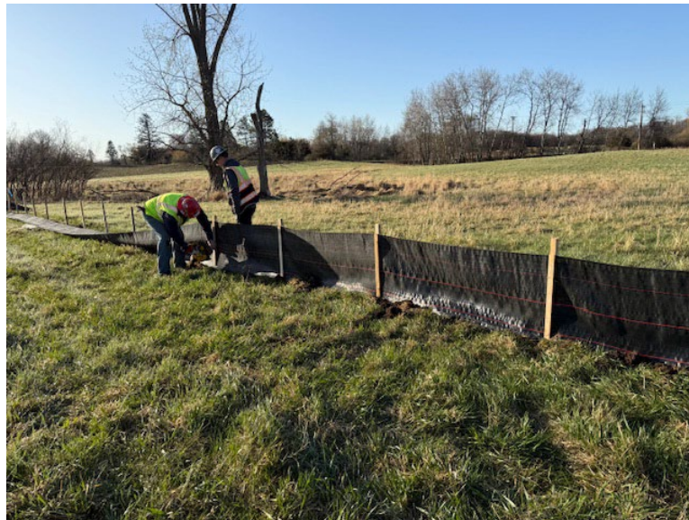
Facing south near MP 1.45, silt fencing installation continued
