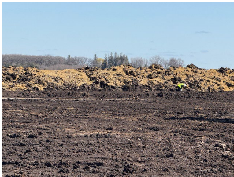
Facing north at MP 34.2, topsoil spoil pile seeded and mulched
