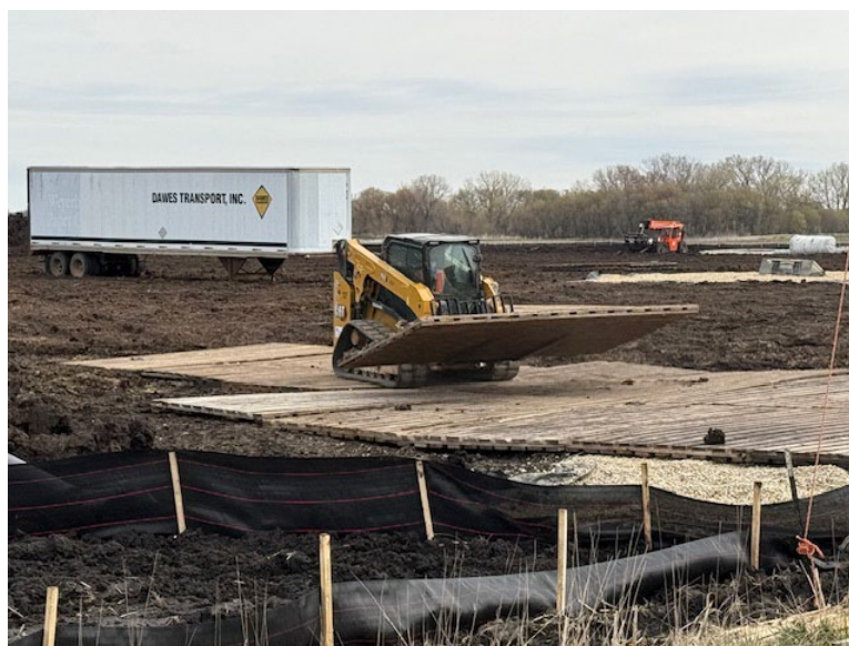
Facing northeast at MP 34.2, K&K installing mats for pipe truck turn-around north of 165th Street
