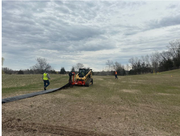
Facing east near MP 1.0, silt fencing installation commenced
